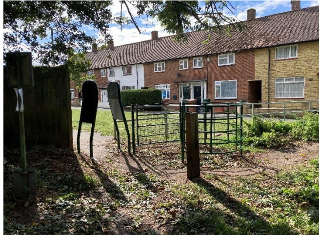
Photo 16: Vehicle barrier improvements were implemented at access points around the site in 2020 with kissing gates and motorbike inhibitors installed.
