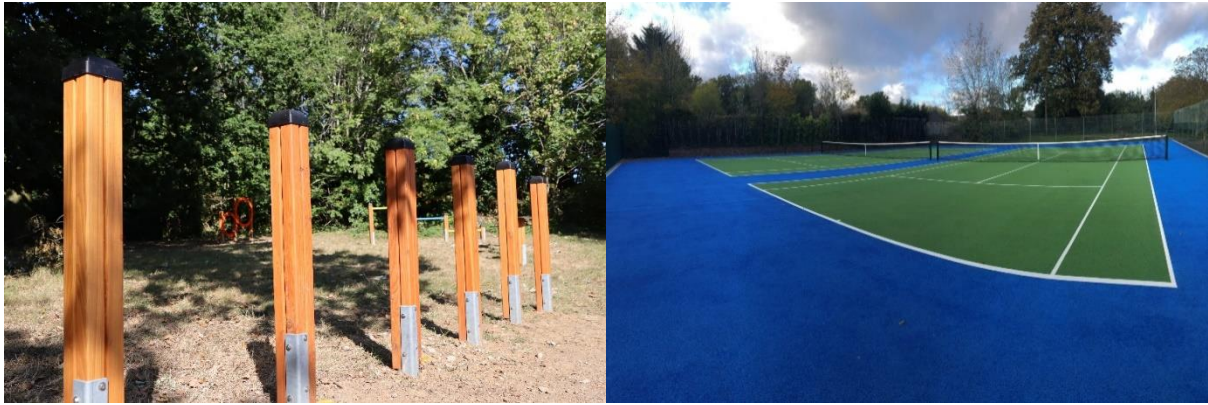
Photo 18: The new dog enrichment area and tennis courts leisure facilities installed on site in 2023.
